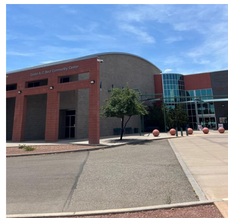
Goelet A.C. Beuf Community Center in Phoenix, Arizona.
